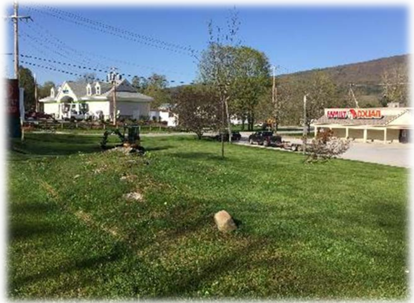
Figure 2: The potential site where sub-surface chambers could be installed as a filtration practice is show in this photo. Only the green space in front of the parking area would be developed for stormwater management.
